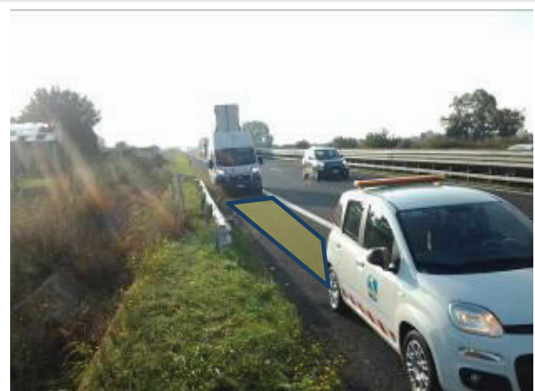
Figure 2: Picture taken during a “punctual inspection” with the safe area protected by the escort vehicle highlighted in yellow. Photo credit: Carlo Polidori).
