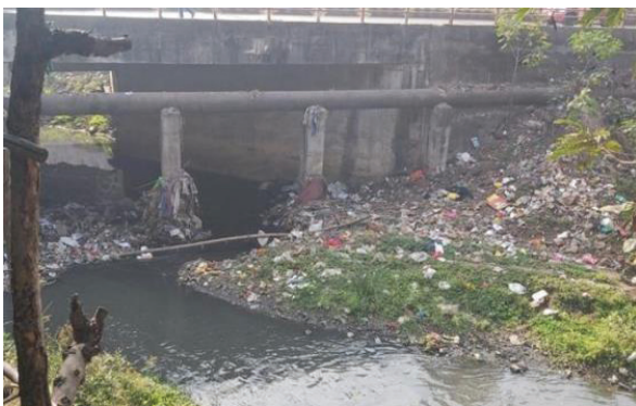
Figure 1: Drainage system near untwadi road.
